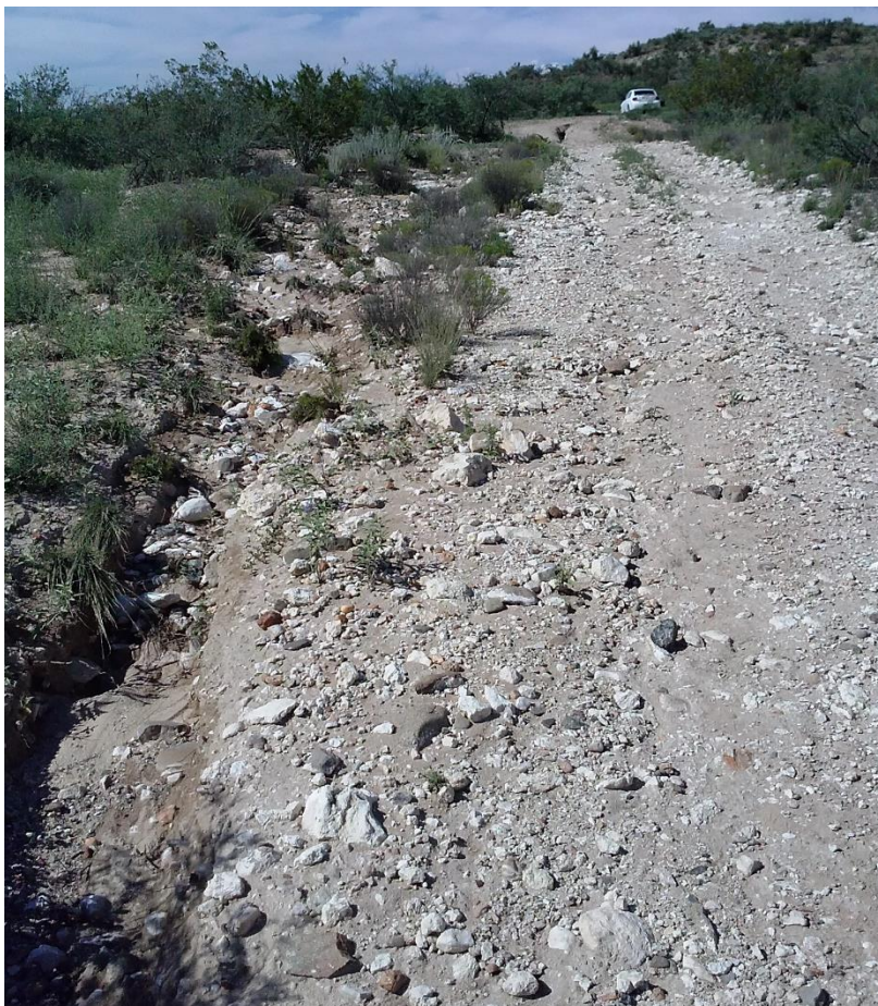
Figure 5.5: Existing Dirt Road Conditions: Drainage on side of road
