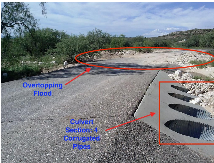
Figure 5.3: Existing Culvert (flow entrance) with Road Overtopping View
